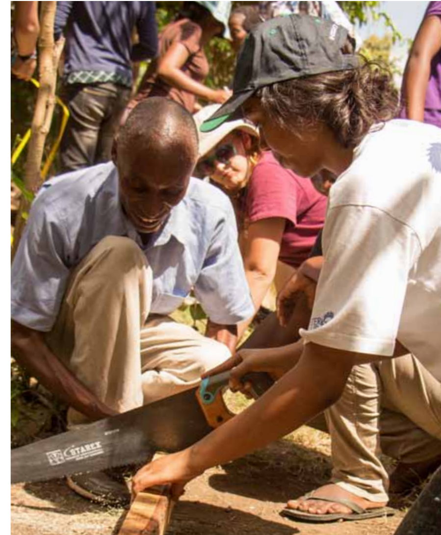
Students from The British School of Beijing, Shunyi, working on a community goat shed project
