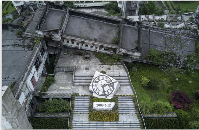
Yingxiu Earthquake Museum and Memorial
